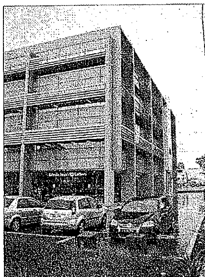
Photograph 5: The existing "CSF" building located to the south-eastern corner of the intersection of Victoria Street and Newton Road.
